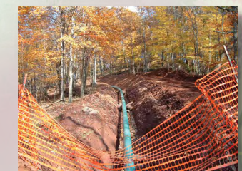
Pipeline in trench
